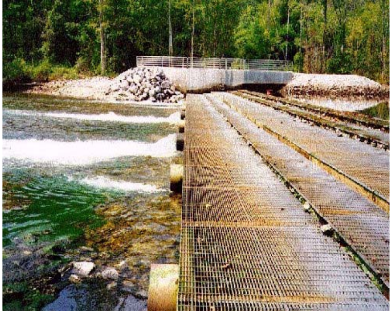
Figure 8. TVA Norris Weir's Stepped Weir Deck
